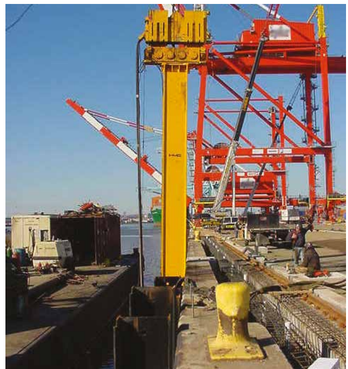
Fig. 12. Installation of AZ below water level with a follower on a vibratory hammer.
