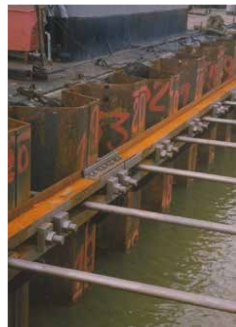
Fig. 6. Conventional anchor solution with tie-rods, walers,...
