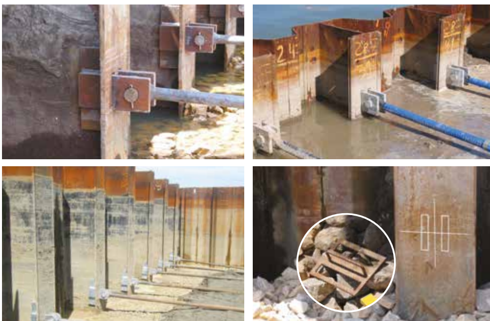
Fig. 5. Installation of the T-connectors at the job-site.
