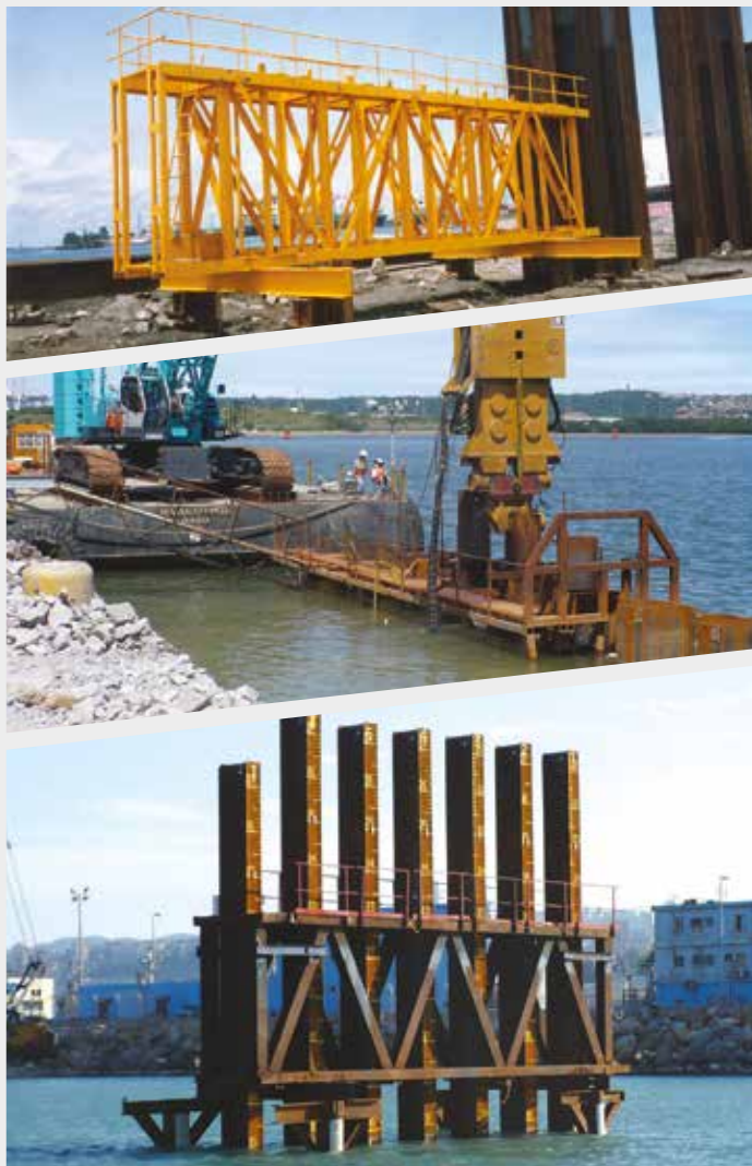
Fig. 9. Driving templates and their support.
